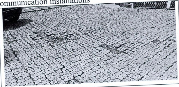
Damaged yard pavement
