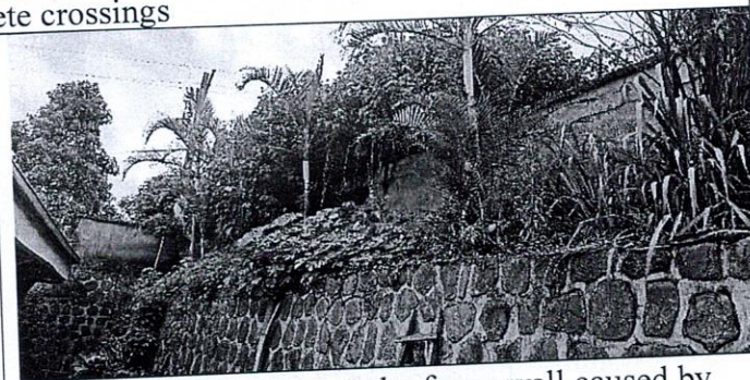
Falling-off plastering on the fence wall caused by overgrown grass on the outside of the wall.
