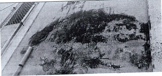
Walls peeling-off especially close to the foundation and toilets
